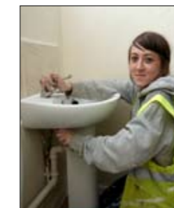
Sammy Earley, apprentice plumber
