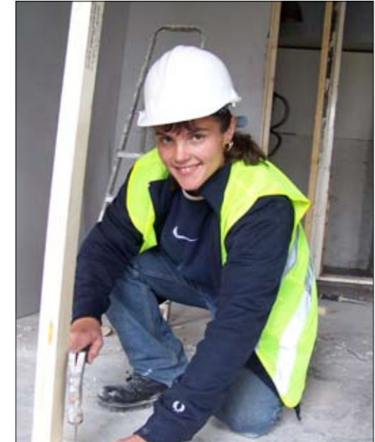
Sarah Hall, NVQ Level 2 apprentice maintenance operations
